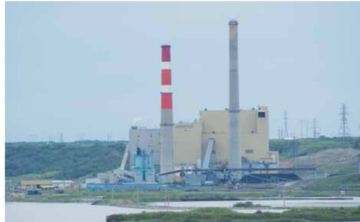
ATCO Power Battle River Coal-Fired Generating Station.
