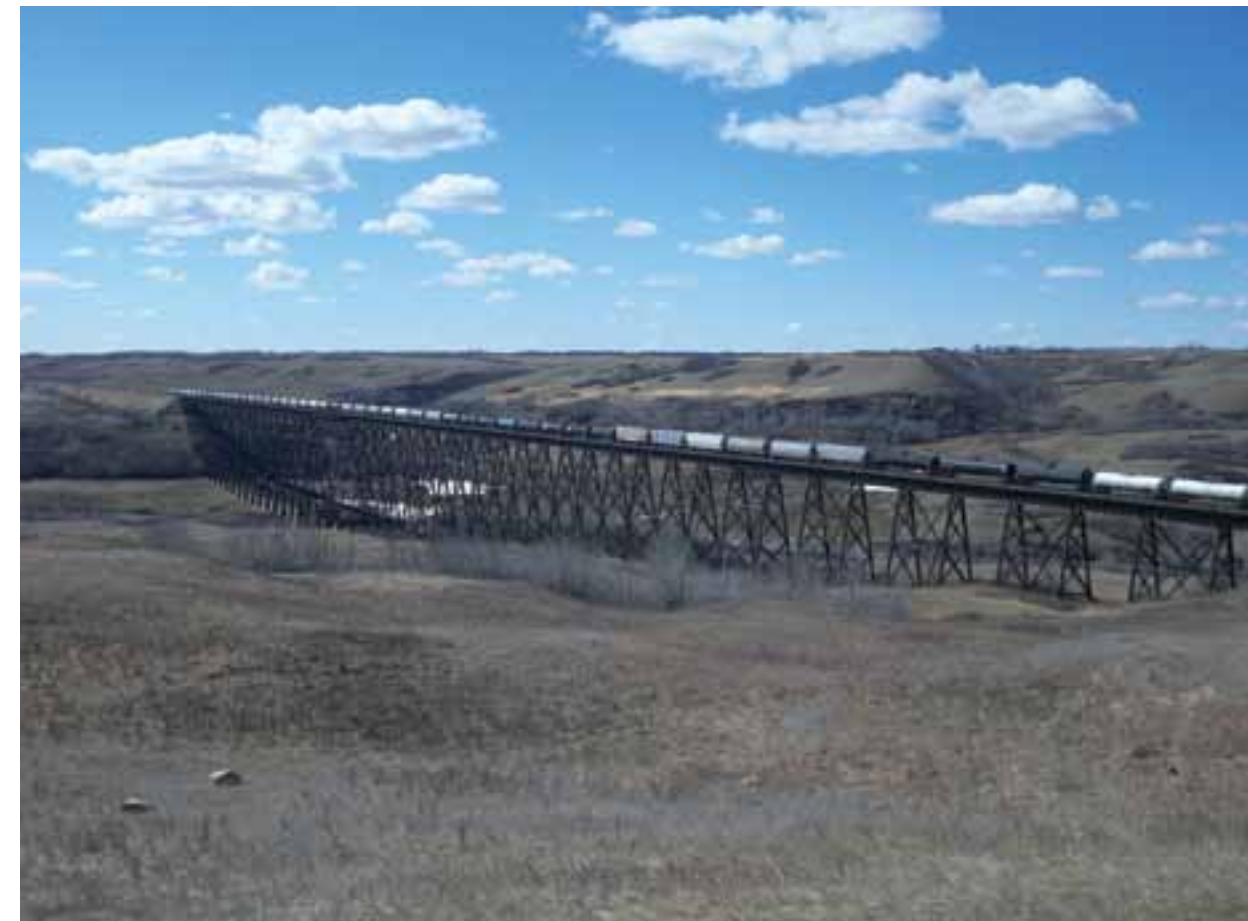
The Battle River Trestle Bridge, located near Wainwright, Alberta.
